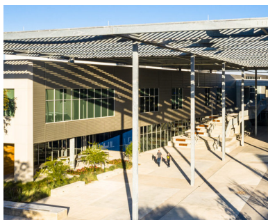
Former shopping mall successfully renovated into a mixed use district at the Highland Mall in Austin, TX.
