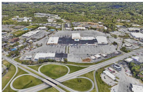
Aerial view of Northgate Mall.
