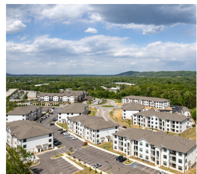
Ridgeview Apartments are a new multifamily development southeast of Northgate Mall.
