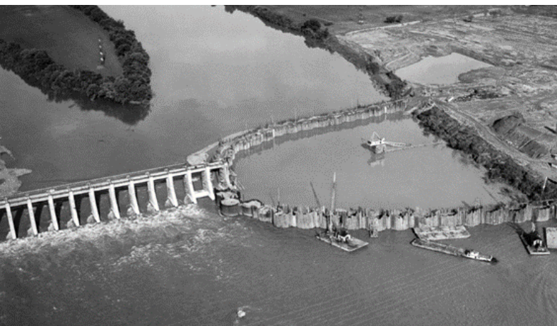
Chickamauga Dam under construction, 1936. Source: Chattanooga History Center
